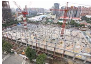
pre-cast Base construction
