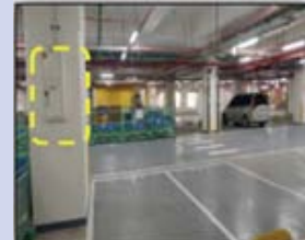
EV Charging Spaces with Power Reserved
