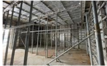
Aluminum Formwork System
