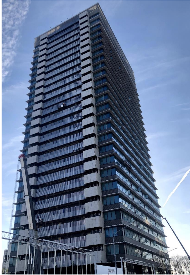
Nangang-Yucheng Commercial Office Construction Project
