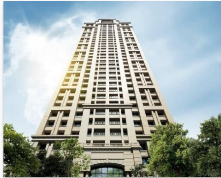
Precast exterior wall
