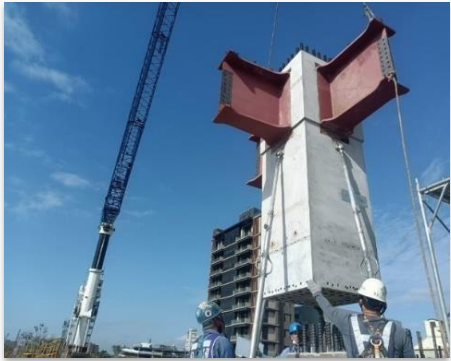
PCS construction method
