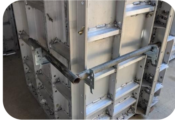
Aluminum Formwork System
