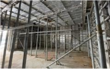
Aluminum Formwork System
