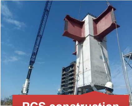
PCS construction method
